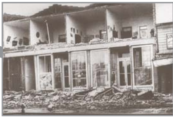
1906—Damage in Healdsburg
