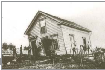
1868—Damage in Hayward
