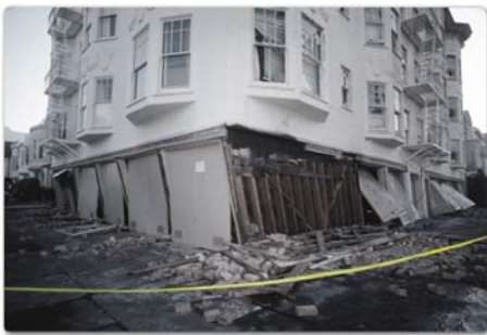
Buildings in the Marina District of San Francisco were badly damaged in the 1989 Loma Prieta earthquake. “Soft story” buildings, typically with parking on ground floor, like the one pictured here, are common throughout the Bay Area and are particularly at risk when exposed to strong shaking. (USGS photo)
